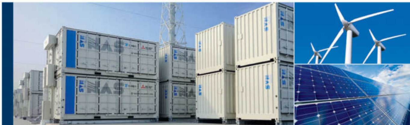
Kyushu Electric Power Co., Inc.'s new 300,000-kilowatt-hour NAS storage array, supplied by NGK Insulators, Ltd., helps balance supply and demand amid Kyushu's surging growth in solar generation. (NAS photo courtesy of Kyushu Electric)
